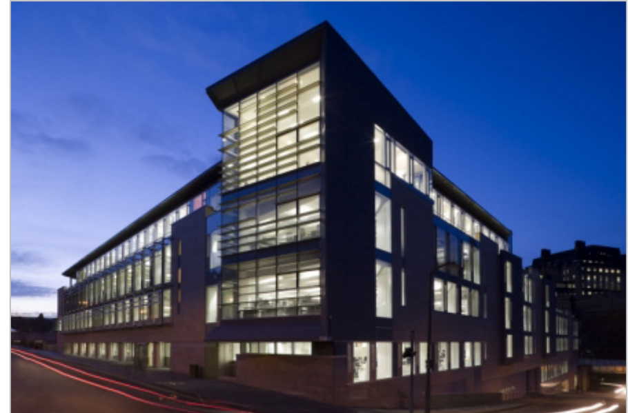
Council headquarters, East Market Street
